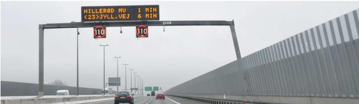
Figure 2 Variable speed signs and variable message signs with text information showing travel times (or other information)
